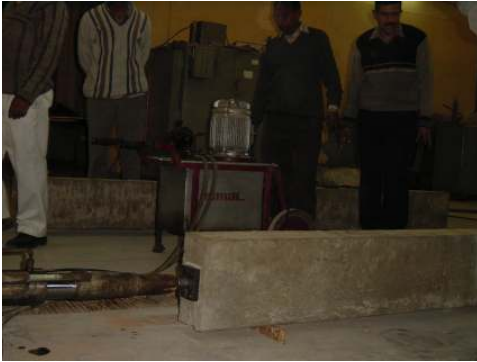
Photo 1: Prestressing Operation in Progress Photo 2: Grouting Operation in Progress
