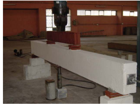
Photo 3: A view of the PSC beam for testing
